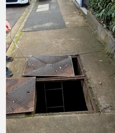
Protection of pits
